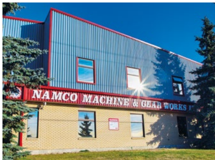
The NAMCO site in Edmonton, Canada. A second location is in Chardon, Ohio/USA.
